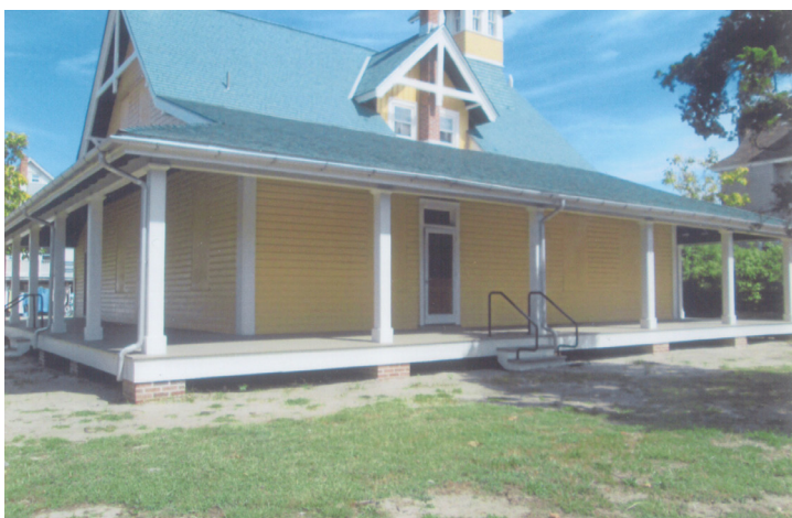
Ocean City Life Saving Station during renovation
