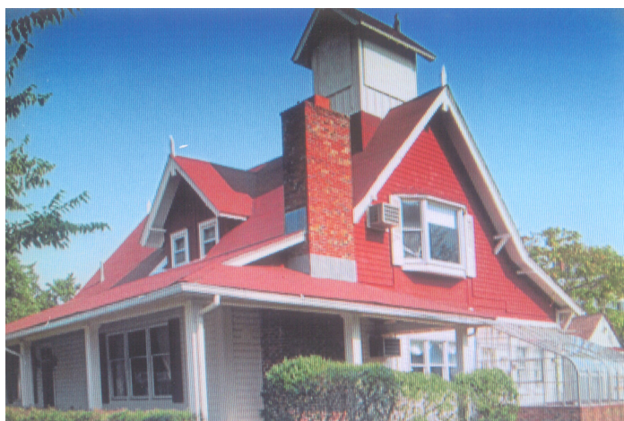
The completed project
